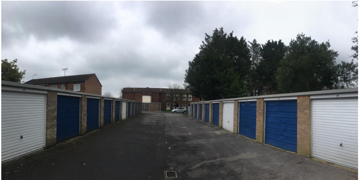
View from the rear of the site looking North West
